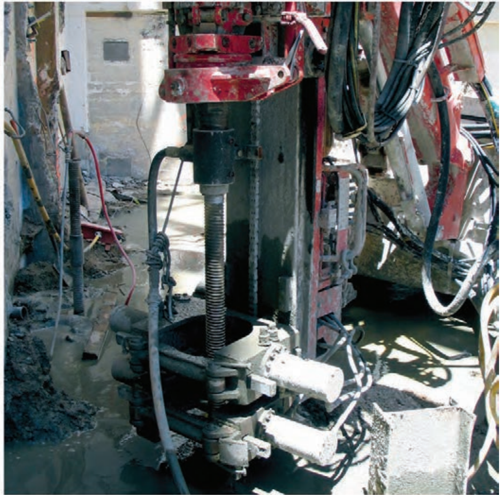
Simultaneous Drilling and Grouting
